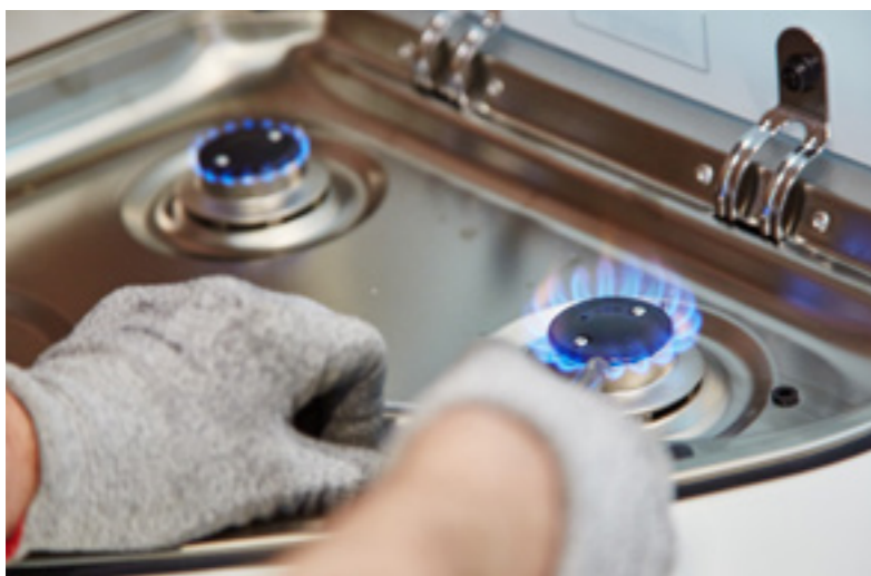
Test on operation of the gas pipes.
